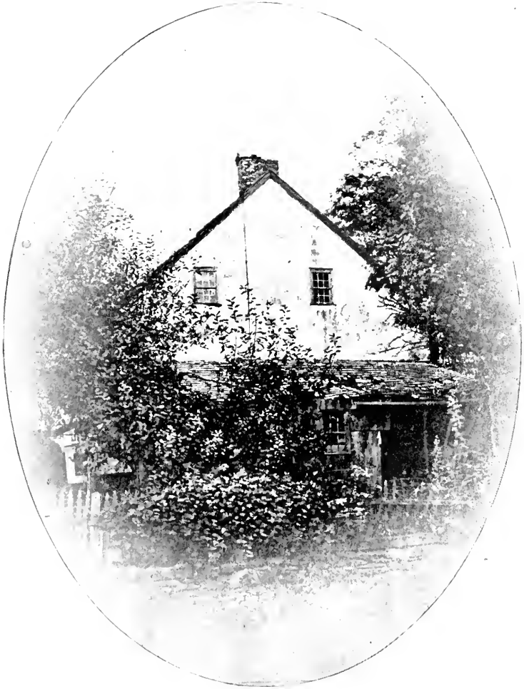
EASTERN GABLE OF THE OLD STONE HOUSE
